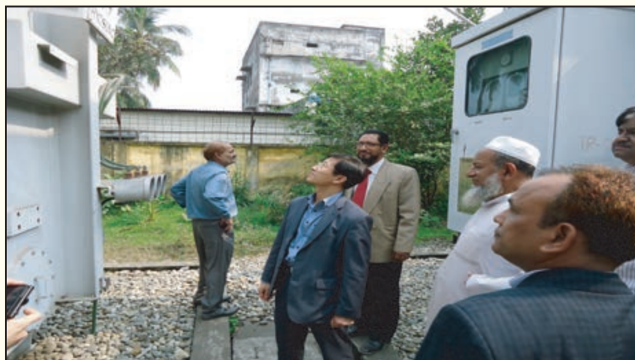
Visiting Khulna City Main 33/11 KV Substation by Korean Delegates
