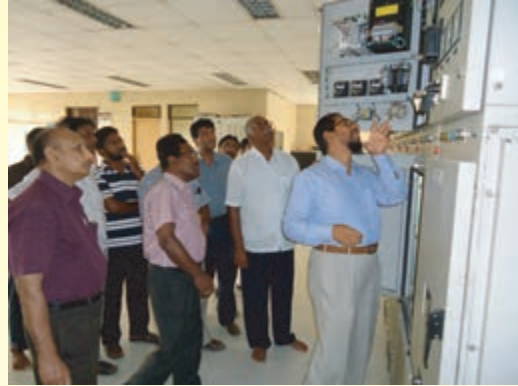
Meherpur 33/11 KV Substation control room Inspection
